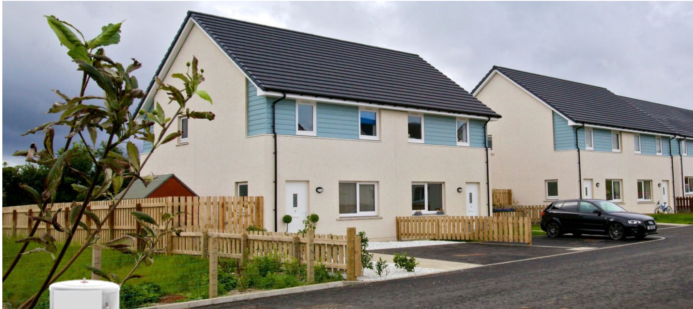
Energy and sustainability strategy focusing on 'Fabric First' and 'low tech' energy options.
